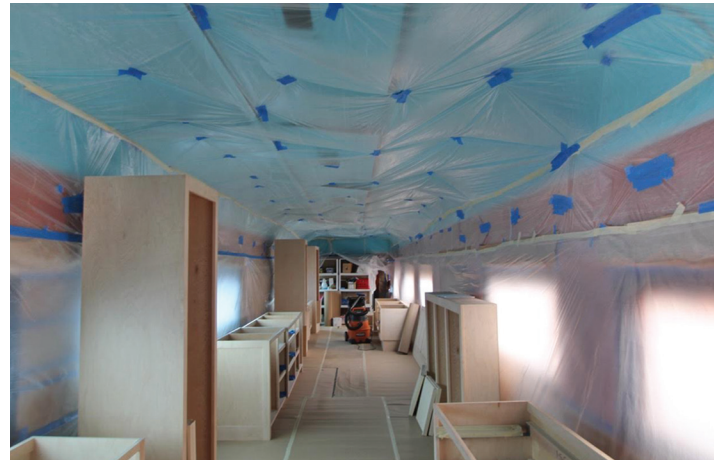
Brand-new wooden cabinetry by carpenter Bill Johnson in the coach-turned-concession-car Cedar Park , where it will serve passengers with snacks, beverages and souvenirs.
